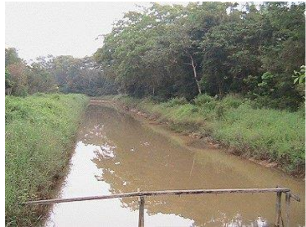
Ditch surrounding lagoons
